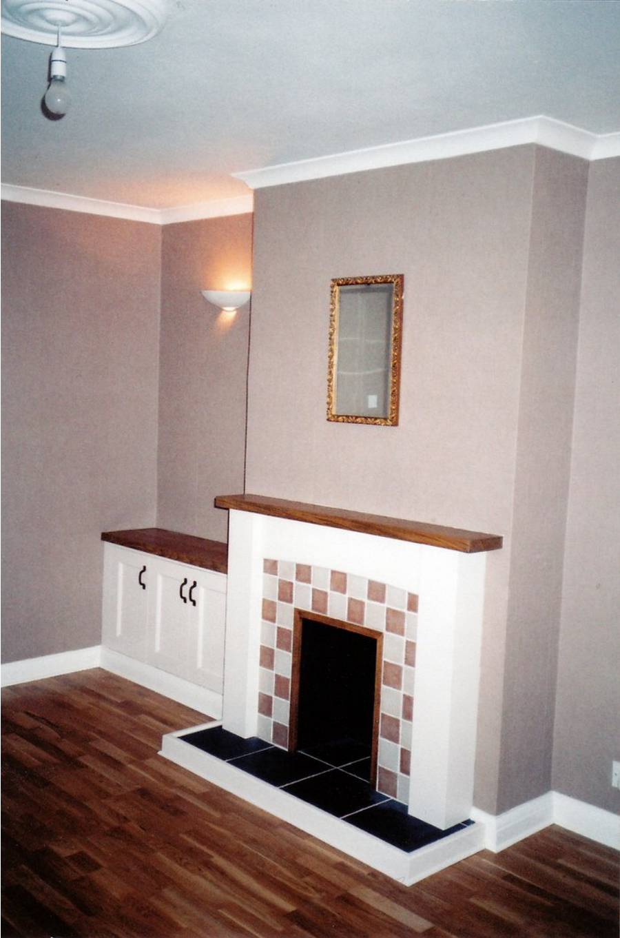
Painted MDF fireplace and alcove cupboards with solid oak mantelpiece and shelf
